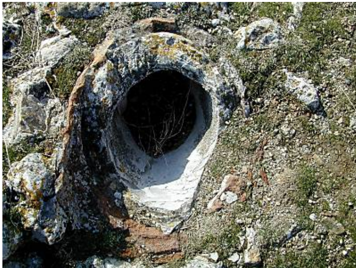
The piped water to Laodicea was lukewarm. It was so rich with calcium that the pipes would block up. So the engineers covered the vents with stones that were removed from time-to-time to permit cleaning.
